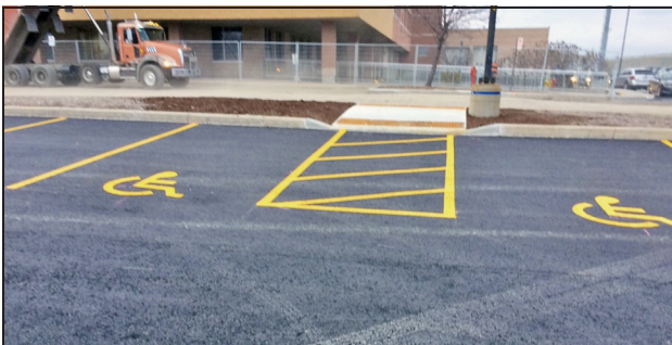
180 Derry Road – Parking Lot
